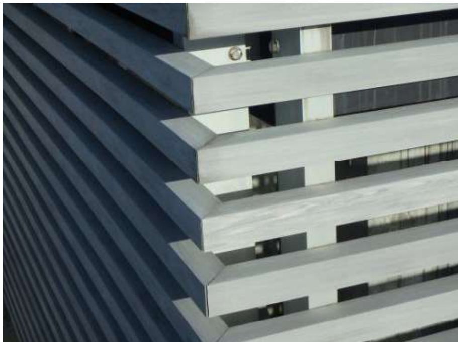
Figure 44 – Close-up of slatted covering corners on the lower portion of the building walls at Pymont Wharves 8 and 9.
