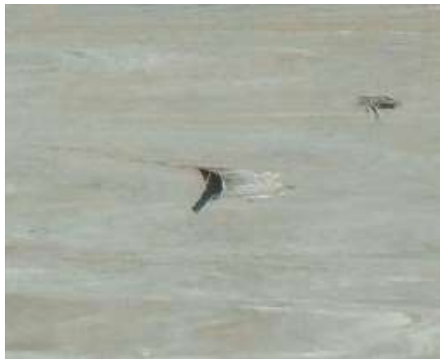
Figure 38 – Detail of (rare instance of) surface peeling in the Wild Life Sydney Zoo Façade
