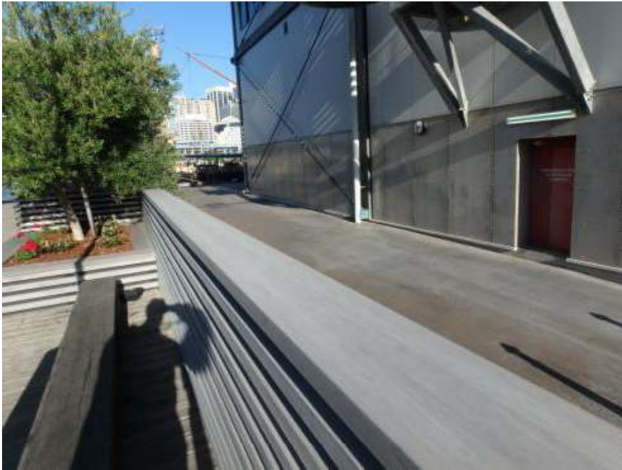
Figure 46 – General view of the planter surrounds and wall feature in front of Pymont Wharves 8 and 9.
